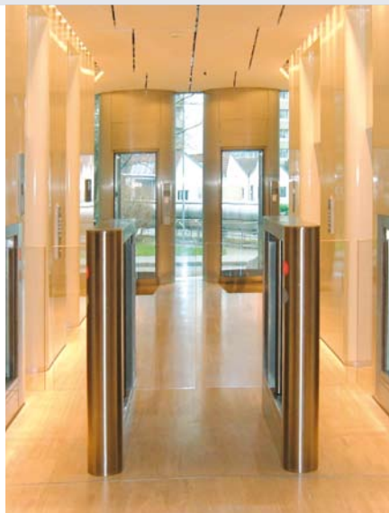
Double access control - sensor barrier with extension unit and Orthos personal interlock system in the background
